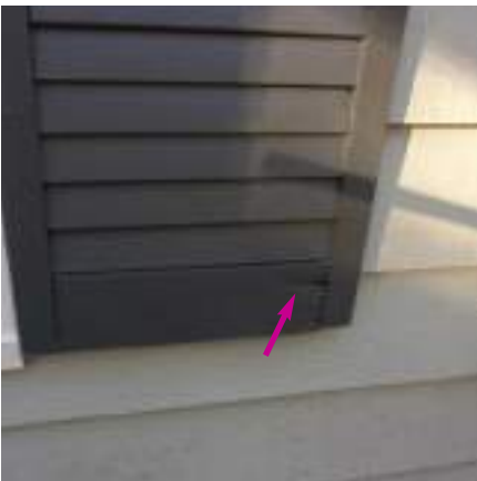
Recommend WDO inspection and any needed repairs. Some wood rot noted including at shutters and at beam in back porch.
