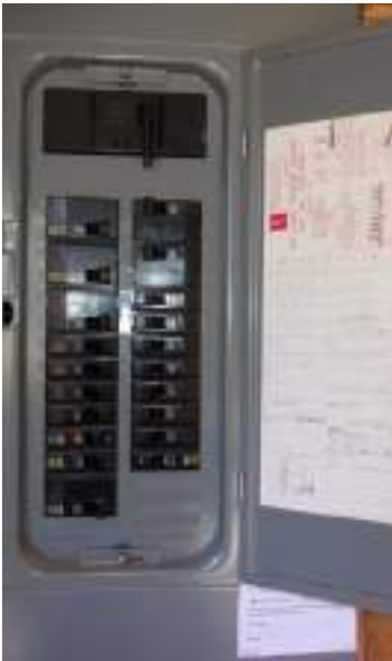
Main electric panel manufactured by Square D was in the garage. 200 amp service was indicated. Copper branch wiring noted. Main shut-off at top of panel.
