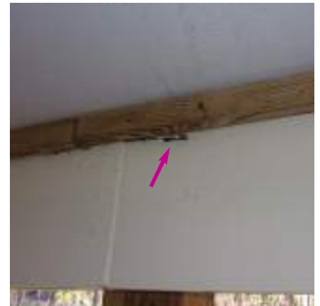
Recommend WDO inspection and any needed repairs. Some wood rot noted including at shutters and at beam in back porch.
