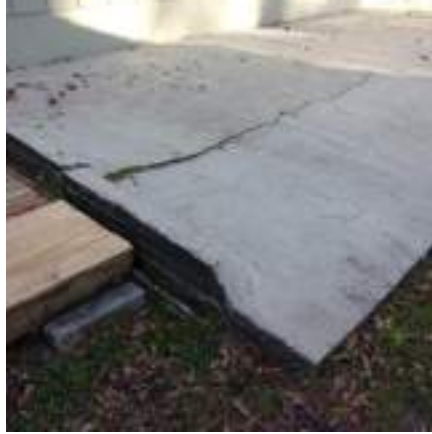
Cracking and settlement noted at driveway in a few locations. Recommend backfilling along edge of driveway and planting ground cover.
