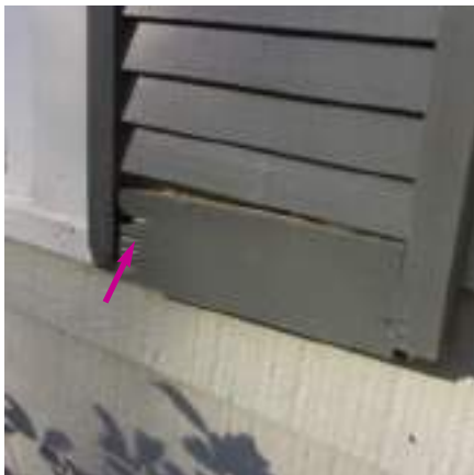
Recommend WDO inspection and any needed repairs. Some wood rot noted including at shutters and at beam in back porch.
