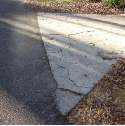
Cracking and settlement noted at driveway in a few locations. Recommend backfilling along edge of driveway and planting ground cover.
